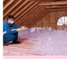
The AttiCat™ Expanding Blown-in Insulation Machine conditions the AttiCat™ Expanding Blown-in PINK FIBERGLAS™ Insulation by breaking it up and fluffing it.
