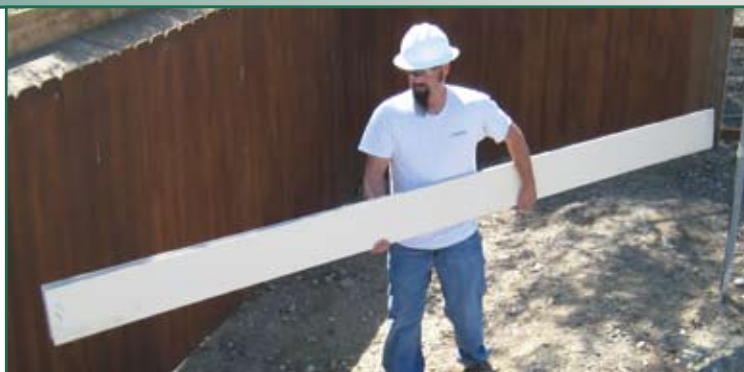
One person should hold planks on edge in the middle with arms spread apart for maximum support of the product
